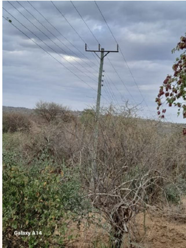
Figure 4: Last mile overhead fiber on KPLC poles
